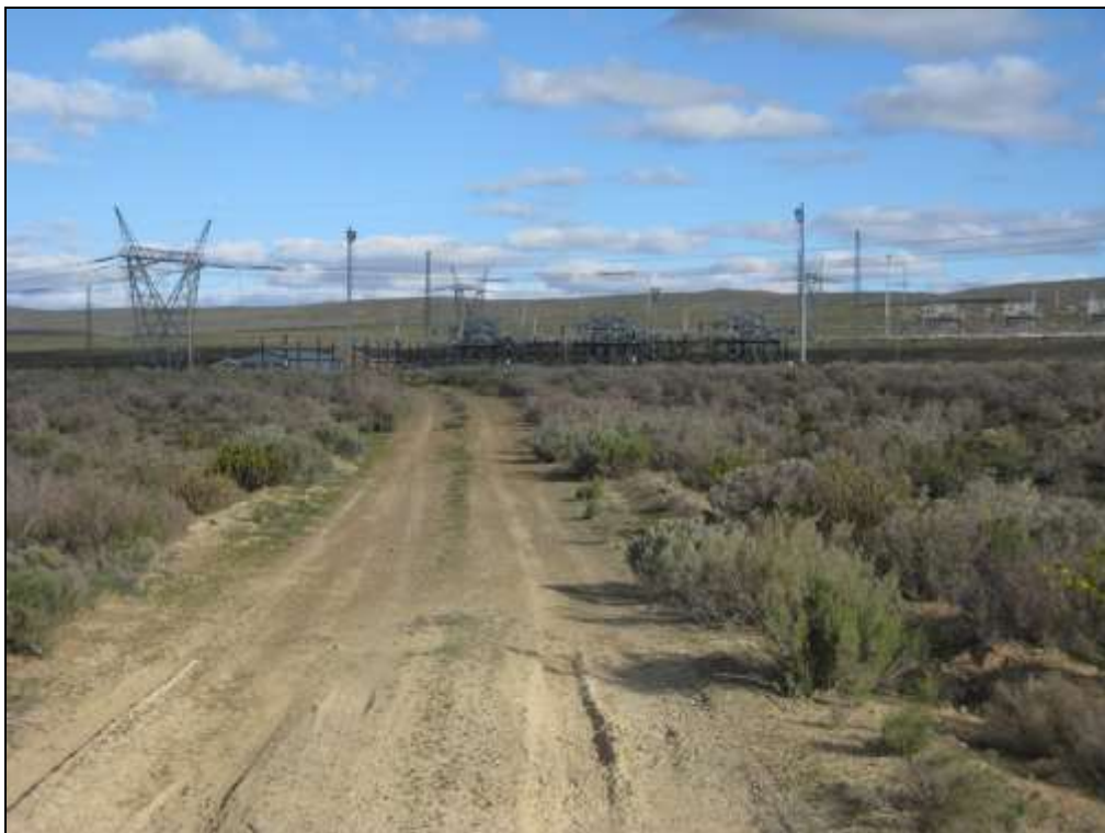
Figure 4. View towards the existing Eskom Komsberg MTS from the west.
